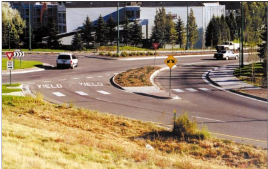
Exhibit 6-41. Example of right-turn bypass lane.
